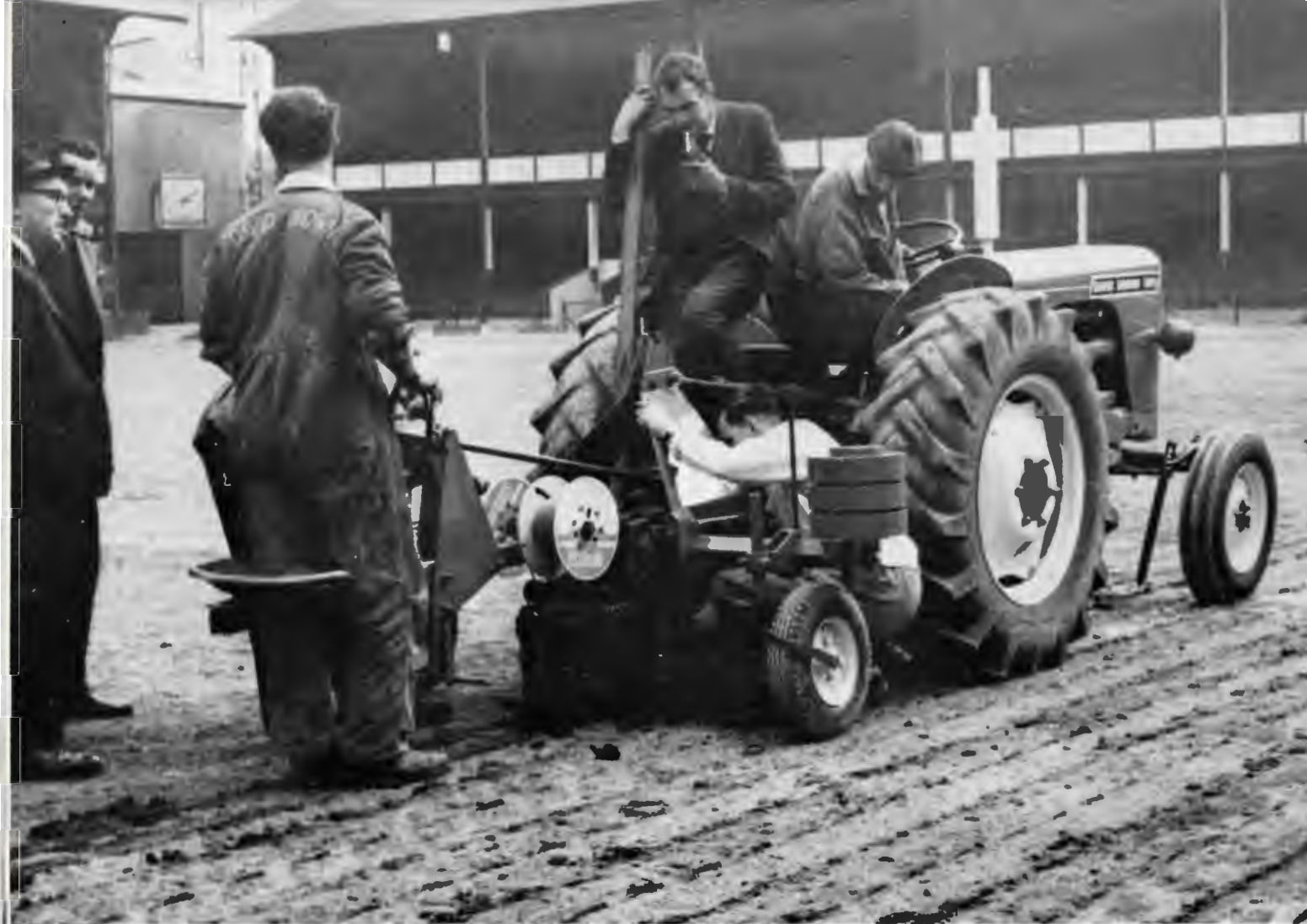
A minor adjustment to the tractor-drawn mole-plough during cable-laying operations at Goodison Park
